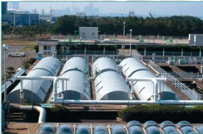
Sewage disposal facility
