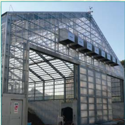
Composting fermentation facility
