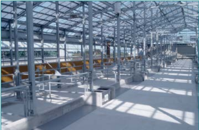
Animal housing* *covered with alternating F-CLEAN™ Clear & F-CLEAN™ Soft Shine
