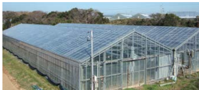
60µm thick F-Clean® installed in the Aichi region of Japan in 1988 (photographed 2009)
