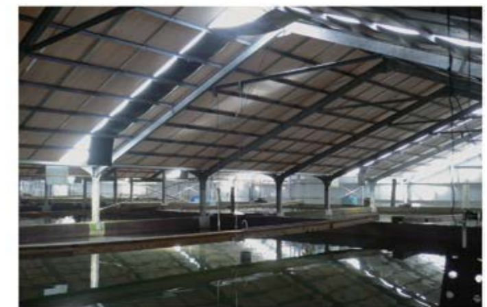
Fish farm facility
