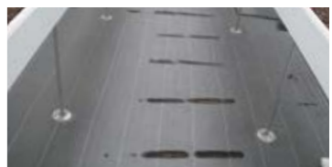
Burned holes in ground sheet
