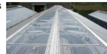
Rainwater on ventilation window
