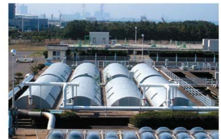
Sewage disposal facility
